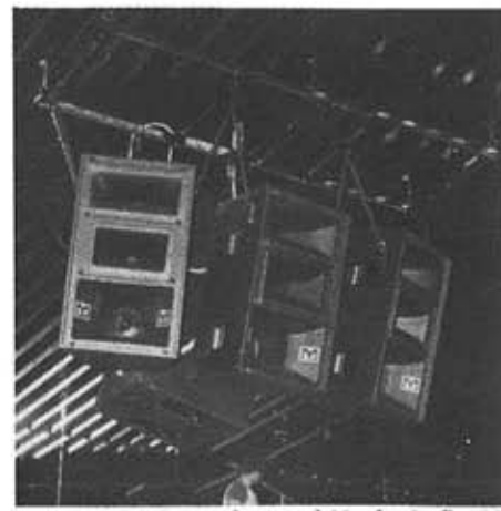
The left-side flown cluster of Martin Audio RS-1203D mid/high cabinets with VRS-800 at rear for stage audience coverage.
