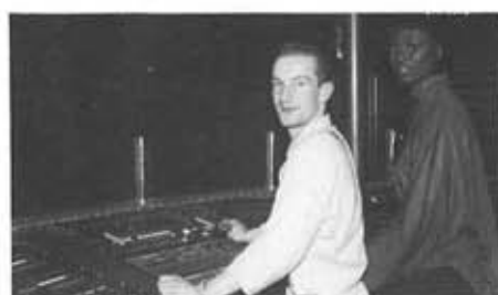
Le Palais' lighting controllers prepare to get the show on the road.
